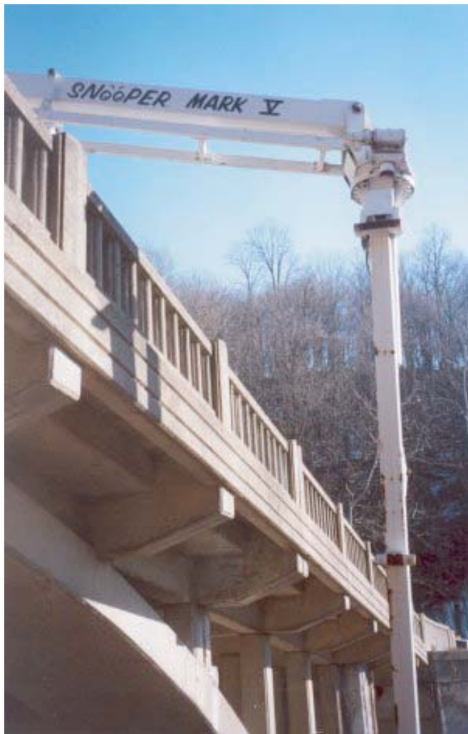
Underbridge inspection "Snooper"
