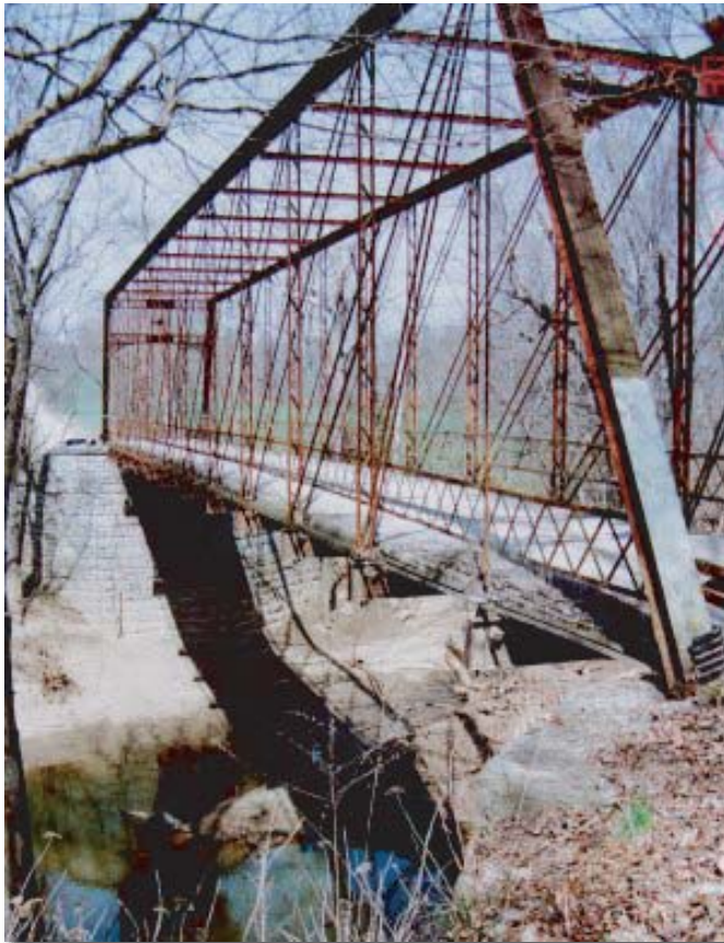
Jefferson County Bridge #30
