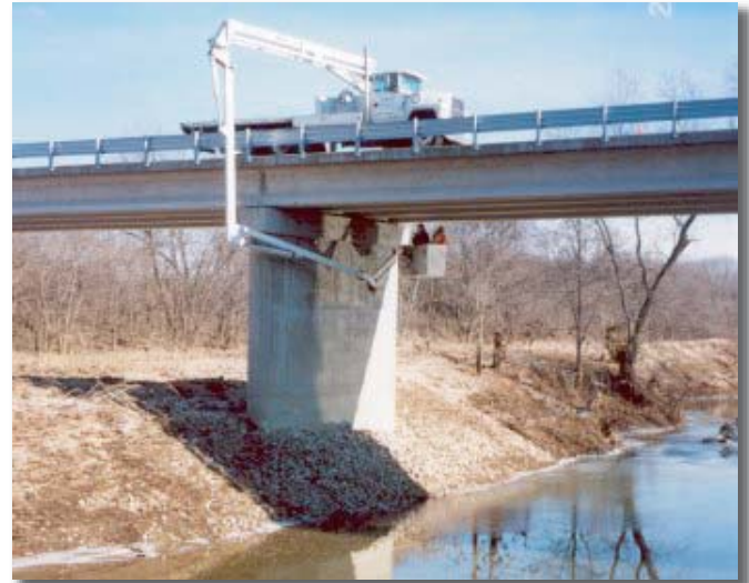
Underbridge Inspection "Snooper"
