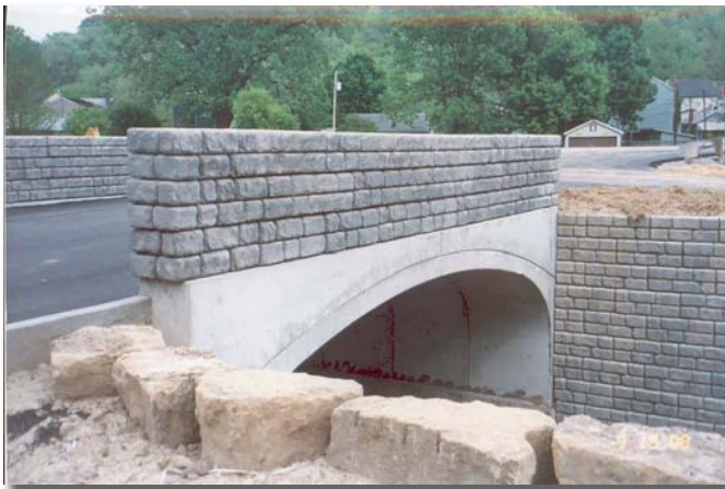
Bridge #4 Jefferson County
