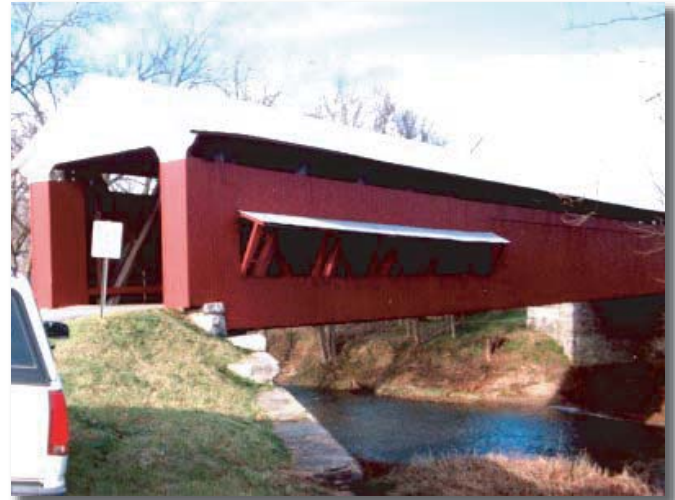
Jennings County Bridge #25
