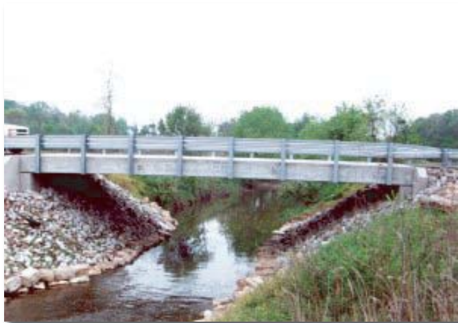
Jennings County Bridge #112
