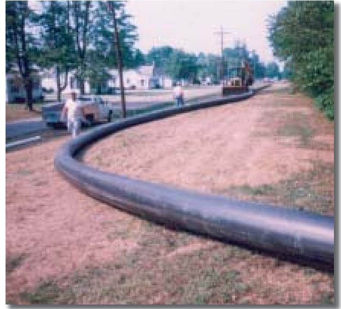
Sanitary Sewer Rehabilitation
