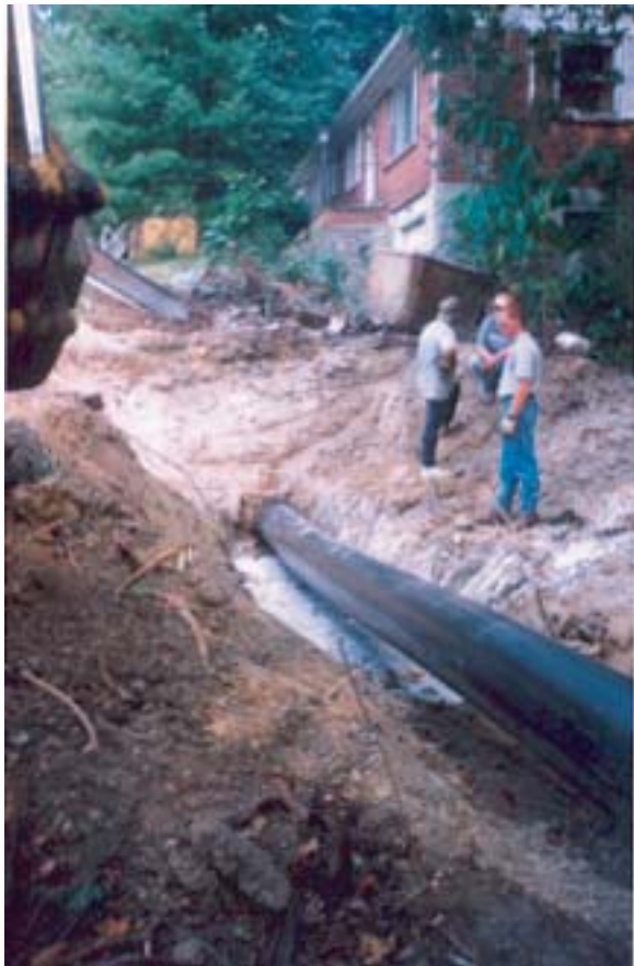
Sanitary Sewer Rehabilitation
